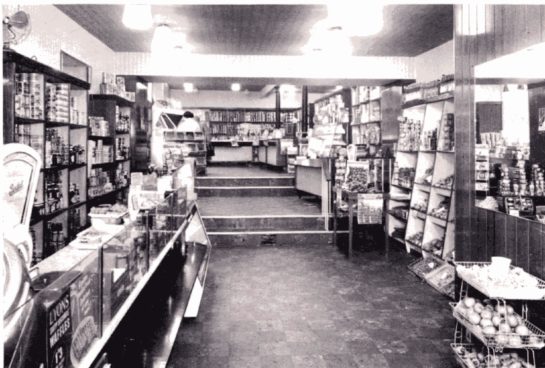
View inside our main branch at 153 High Street, Dunfermline. Telephone 1908.
